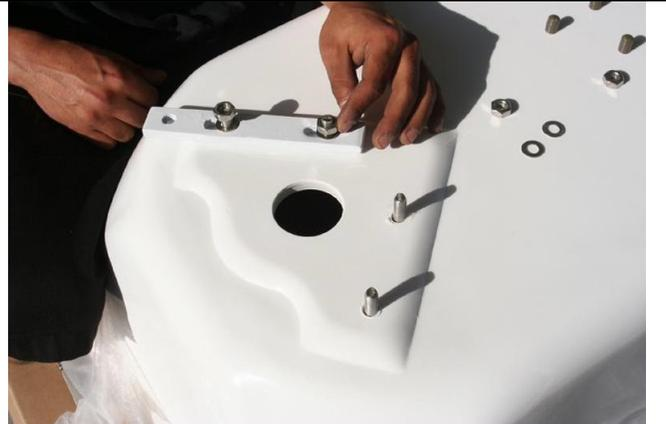
4. Place the claw foot in position. Hold the claw foot in position against the tub as you screw in the foot fixing bolt.
