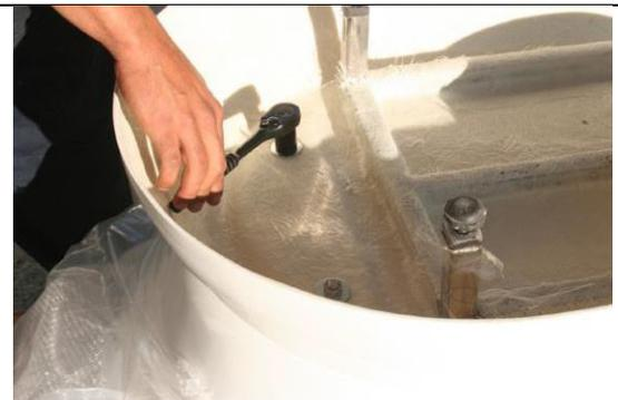
8. Turn the tub upright and position it over the drilled fixing holes. Use a screw or bolt to suit your floor material.
