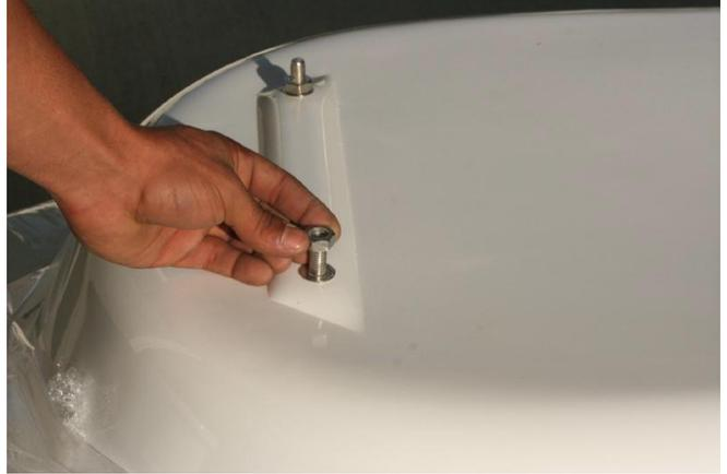
3. Loosely attach the bars to the base of the tub. Don't tighten fully as you will need to adjust later. If your tub is double ended, it will only have two straight bars, no V bars as shown in this generic photo.
